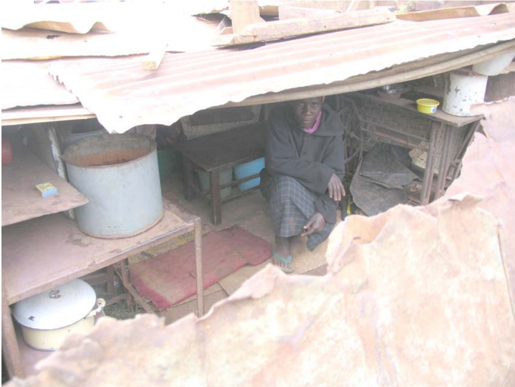
“Revai R.” and her family had to assemble this shelter from pieces of metal and wood in Harare, after their brick house was destroyed during Operation Murabatsvina. © 2005 Human Rights Watch
